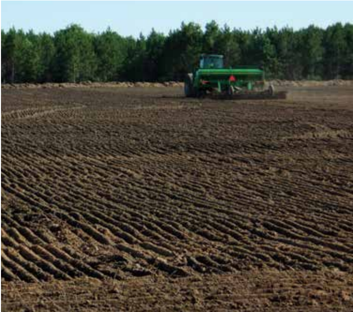
Leveling and preparing the site for grass seeding.
