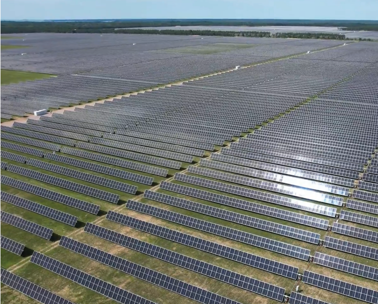
Under the project's bifacial panels are native grasses and seed mixes. Now producing clean energy for the grid, the solar panels track the sun throughout the day.
