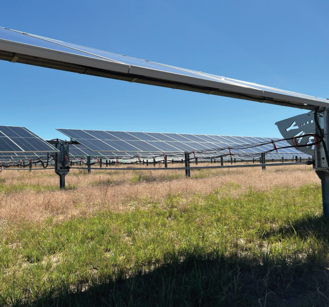
Under the project's bifacial panels are native grasses and seed mixes. Now producing clean energy for the grid, the solar panels track the sun throughout the day.
