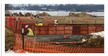
The project substation will be located along W. Pomeroy Road at the northwest corner of the solar arrays and will, via transmission lines, connect the array to the electrical grid. The substation control house foundation was poured. The control house – about the size of a trailer – is a weatherproof building for additional equipment, repairs, or testing necessary. The substation is nearly 30% complete.
