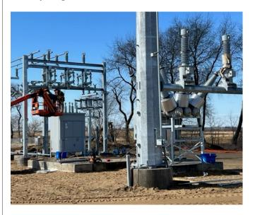
The on-site project substation is 75% complete. The transformer that steps up the substation's output voltage was installed last month and will undergo testing over the next few weeks.
