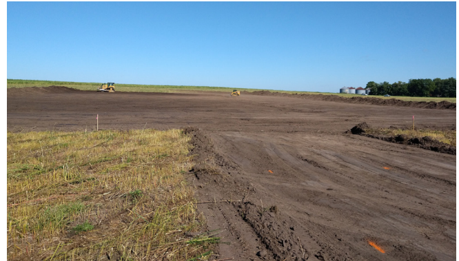
Grading has begun at the Paddock Solar Project.
