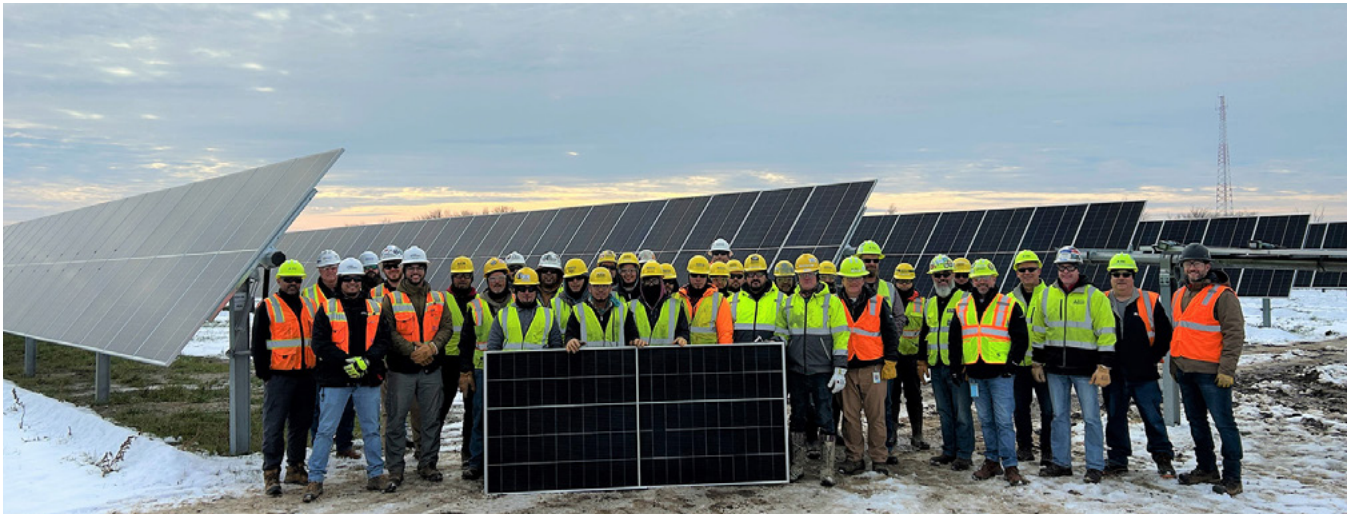
The Beaver Dam Solar Project team poses with the final panel installed as part of our Wisconsin solar program
