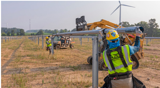
◀ Team members install a torque tube for the Springfield Solar Project tracker system.
