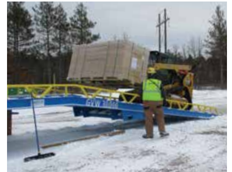
Unloading solar panels from the delivery truck
