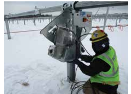
Connecting the tracking system
